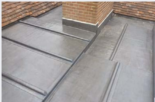
Lead and chimney work
