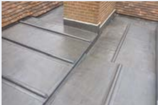
Lead and chimney work
