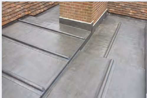
Lead and chimney work
