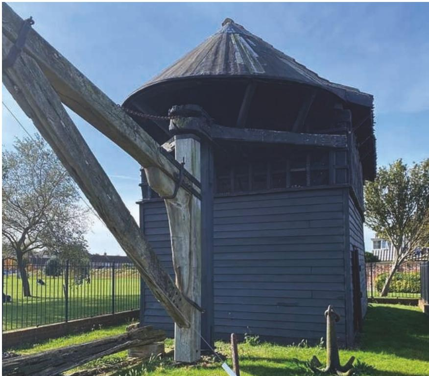
**T**he unique machine was built, possibly as early as 1667, on the docks at Harwich to assist in loading and unloading cargo. Two 16ft high wheels set four feet apart on an axle were worked by a man ‘walking’ inside each one to make them turn and operate a jib, which protruded over the dock from the wooden structure housing the wheels.
