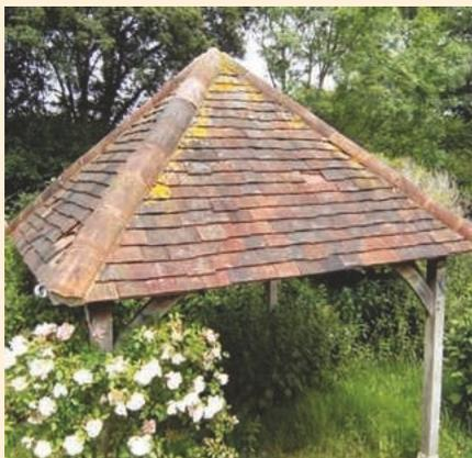
Peg tiles retain their popularity due to the simplicity with which they have been made and fired and for aesthetic reasons which result in subtle variations which are not repeated by modern manufacturing methods.
