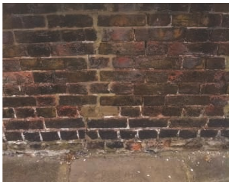
BEFORE: Cement repair to pavement level brickwork on a house in Sandwich
