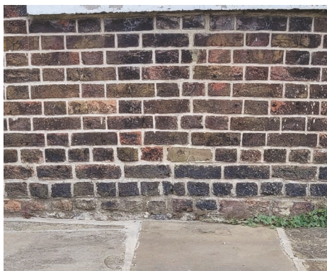
AFTER: The cement has been raked out, replaced with lime mortar and finished with a brushed heritage joint.
