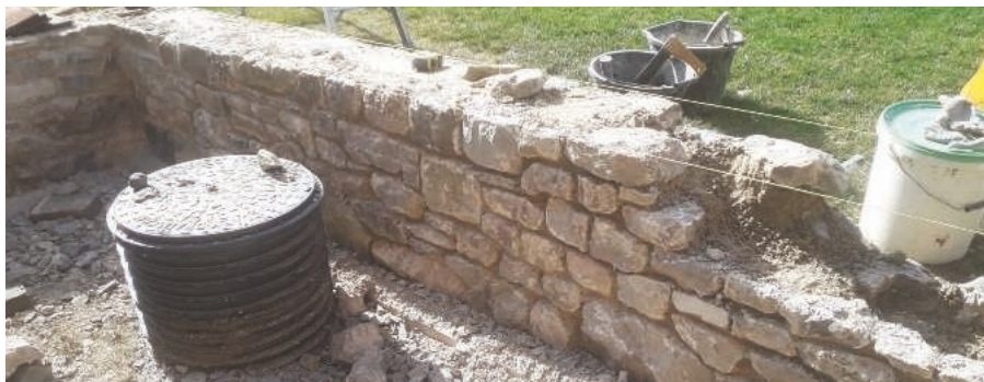
Bloors Manor dwarf wall under construction
