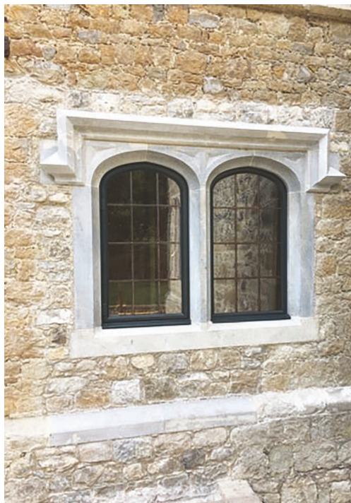
Bloors Manor detail showing the completed double light window replacing the doorway
