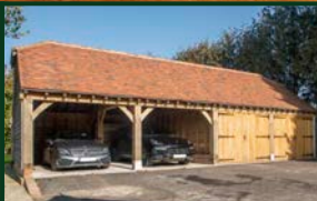
OAK FRAMED BUILDINGS
